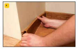
Montaÿ dekoracyjnej czÿÿci listwy poprzez wsuniÿcie jej w naroÿnik. Installation of the decorative part of the plinth by inserting it into the corner. Fixing of the decorative skirting board part by inserting into the corner.
