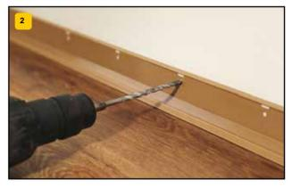
Mounting the skirting board using quick-assembly pins or glue. Mounting the skirting board with quick fixing dowels or glue. Skirting board fixing with fast fixing studs or glue.
