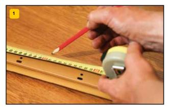
Accurate measurement and cutting of the skirting board to size. Precise measurement and cutting of skirting boards to size. Exact measurement and trimming the skirting board to the desired dimensions.
