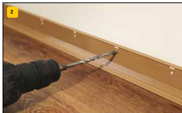
Mounting the skirting board using quick-assembly pins or glue.
