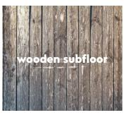
Check the floor for insect infestations. Make sure the subfloor is levelled and screw down any loose sections firmly. Wooden subfloors should always have access to air and should be ventilated at the edges. If there is any moisture in the wood-based subfloor or there is no proper moisture barrier below the wood-based subfloor, it must be removed first.
