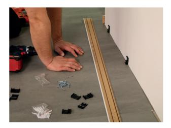
You should use filler twine as a basis for filling expansion joints. Profiles, doorstops and suchlike should not be screwed through the floor covering into the subfloor.
