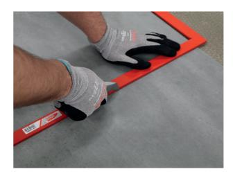
The remaining piece cut off from the last tile in the first row may serve as the first tile in the second row provided it is at least 30 cm long. Always stagger the end joints from row to row, a minimum of 30 cm apart.
